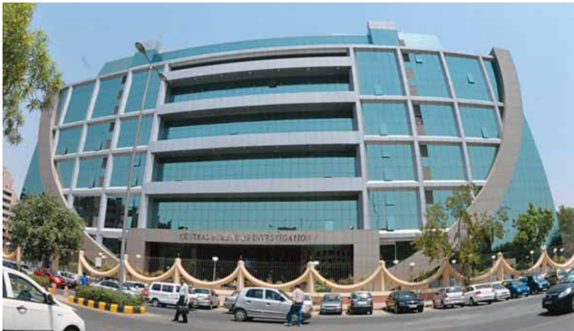
New Green Building - Central Bureau of Investigation Office, New Delhi
