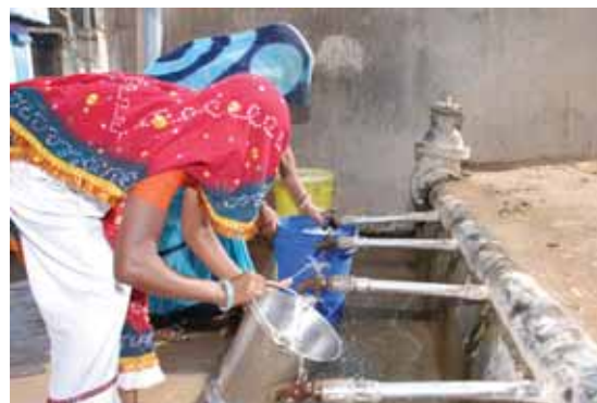
Drinking Water Supply under Bharat Nirman
