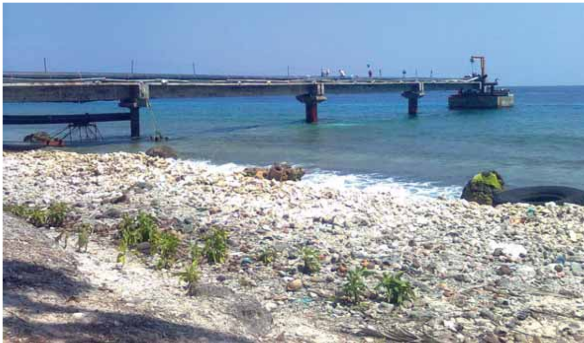
Desalination plant, Minicoy, Lakshadweep
